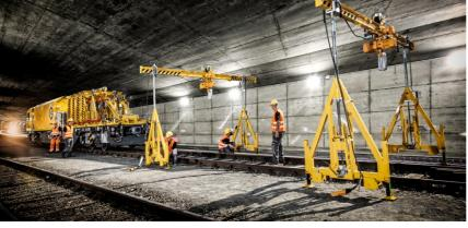
An automatic loading/unloading system moves the gantries over the buffer beam and places them on the track [Fig. 2]. The
