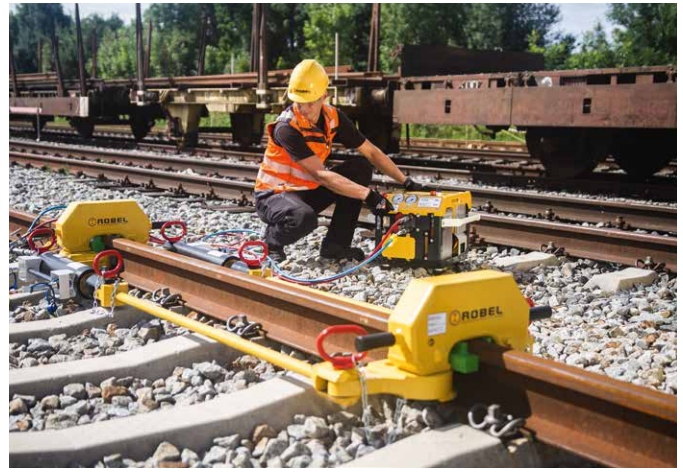
Fig. 7: A battery-operated high-pressure hydraulic power pack supplies energy to the rail stressor and the weld trimmer.
