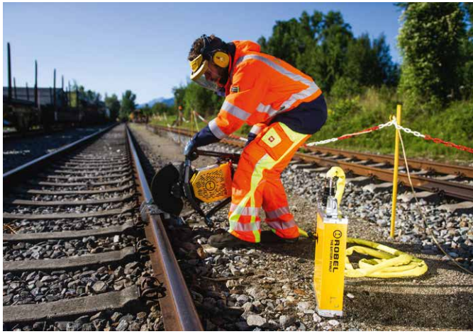
Fig. 6: Driven by a 2300 Wh battery, the electric rail cutter manages up to 20 cuts on a UIC60 rail.
