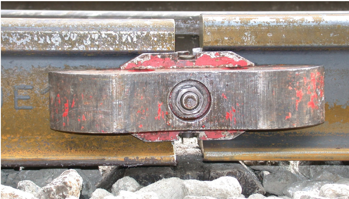
Fig. 6: The use of connecting straps makes it possible to unload rails in longitudinal direction without causing any damage.
