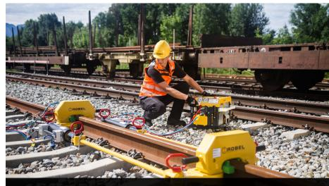
Picture 2: One battery-powered high-pressure hydraulic aggregate operates two machines: the rail stressor and weld trimmer © Robel
